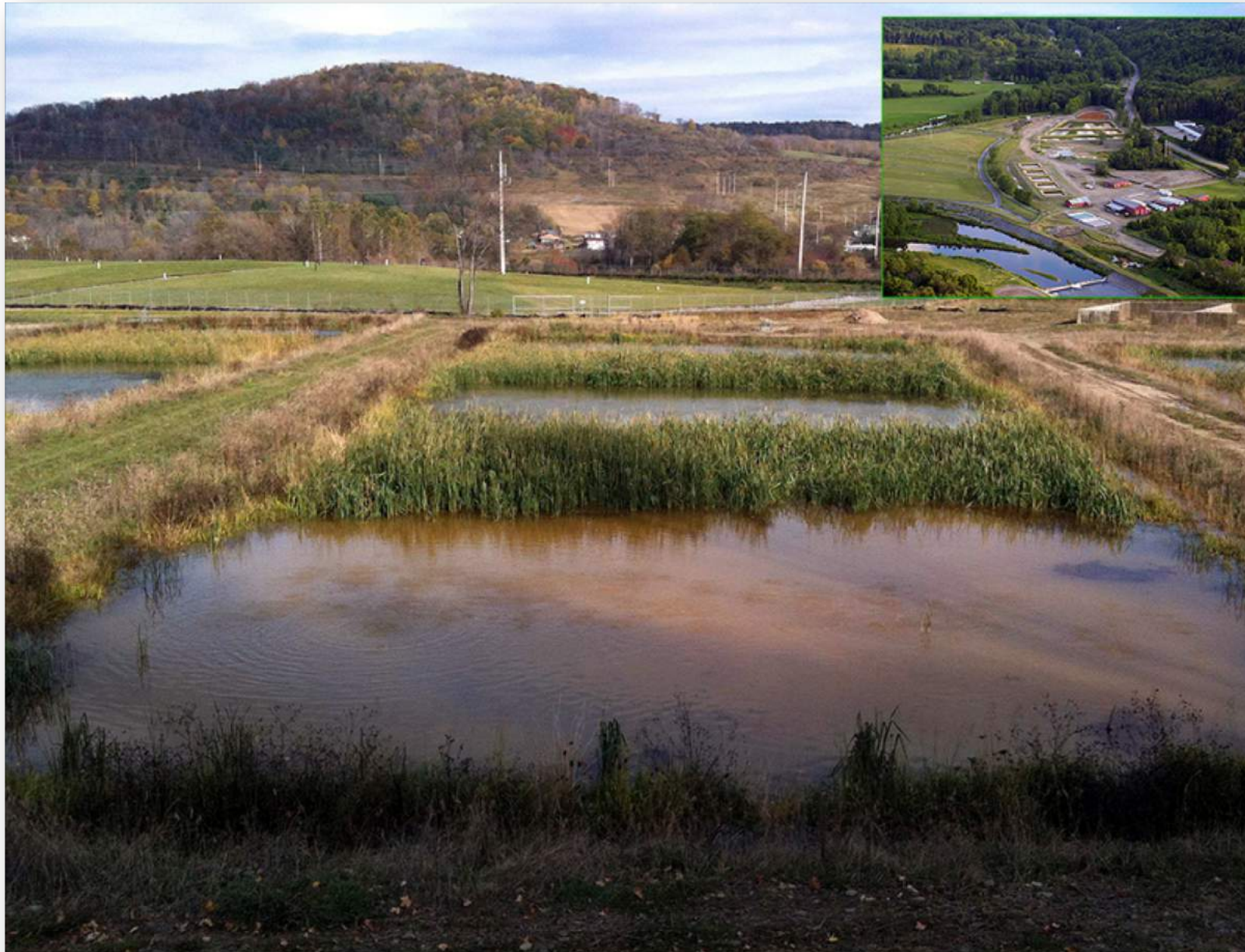
ARCO Refinery (Wellsville, New York)
